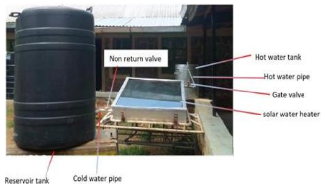
Fig. 2: Layout of flat plate solar water heating system
